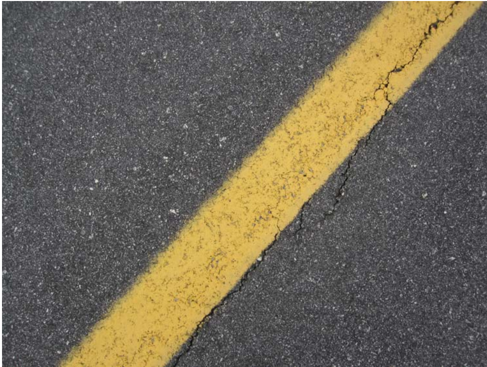
TAJK-10. Satisfactory Paint.
