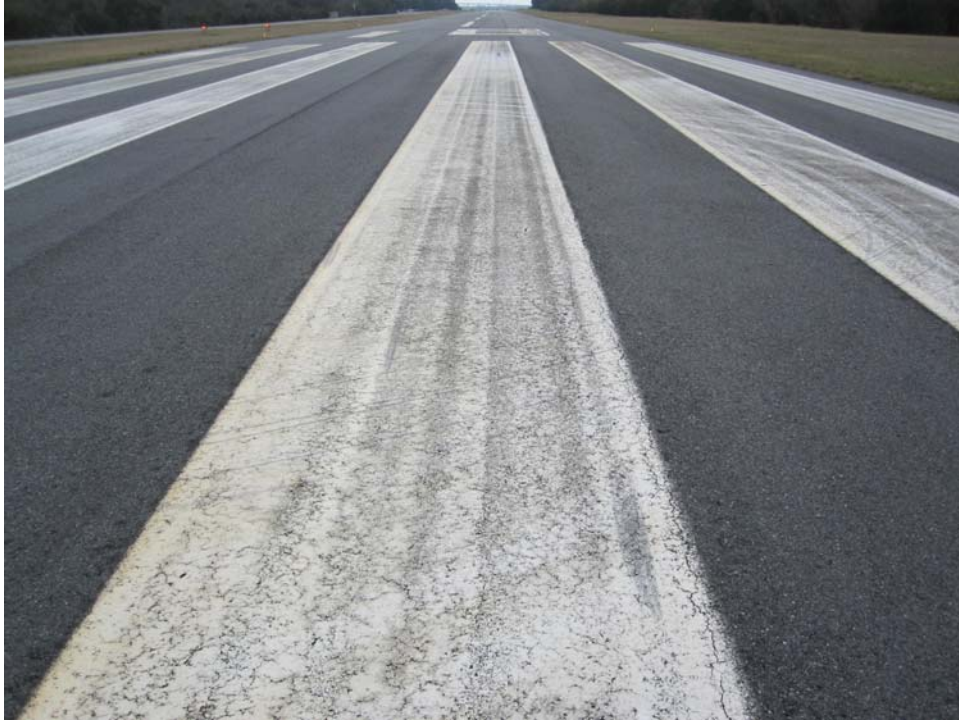
R1836JK-10. Satisfactory Paint.
